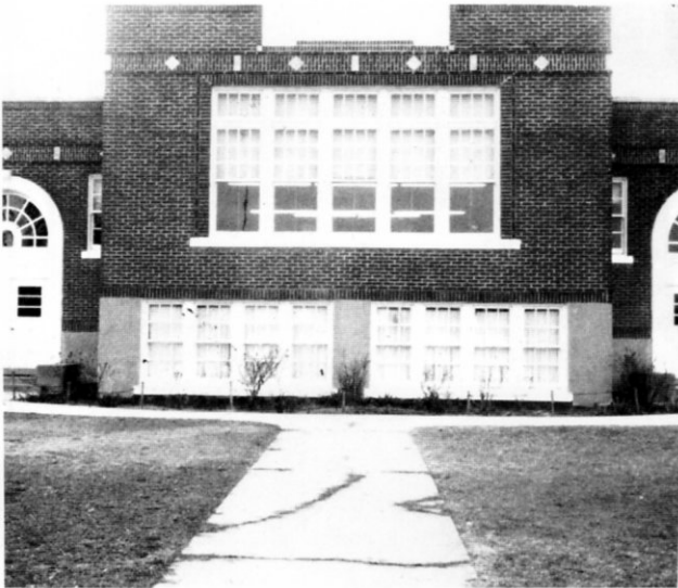
This became known as the ninth grade building and also the place where Coach Robins had his office and also ninth grade lockers are here.
