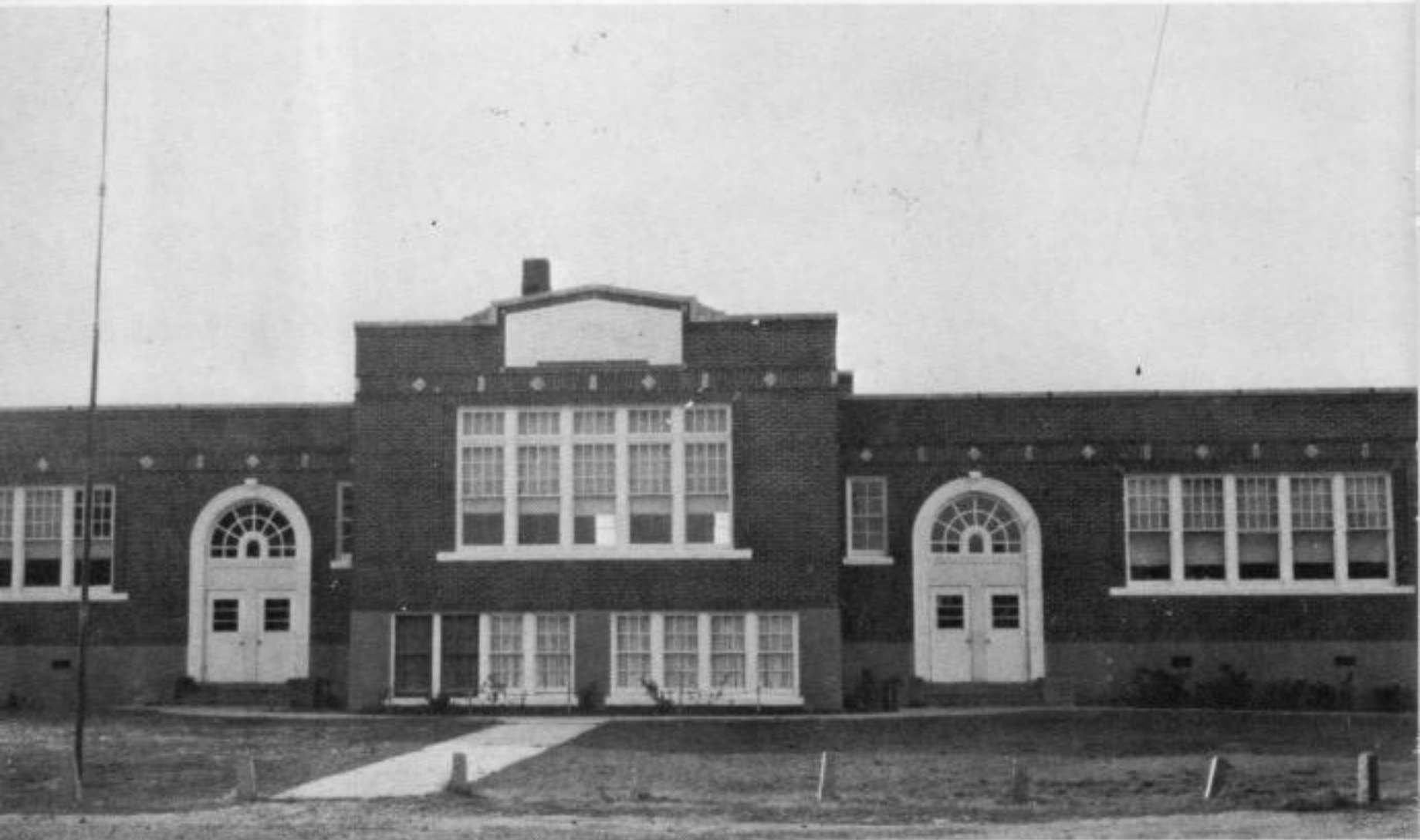
Our Oldest Building
